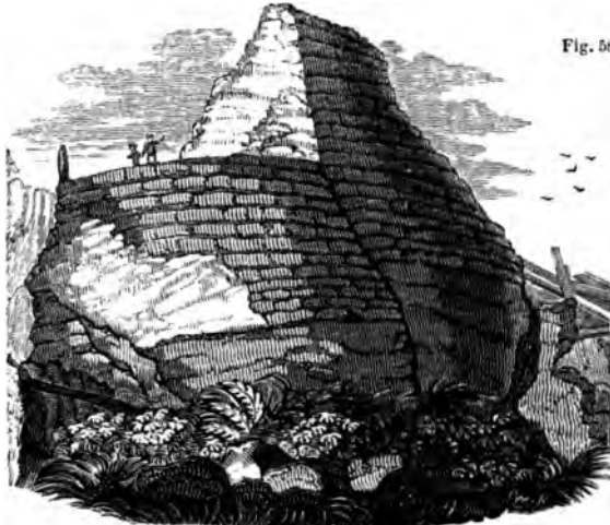
Shift or "fault" in the Round Tower of Terranuova in Calabria, occasioned by the earthquake of 1783.
